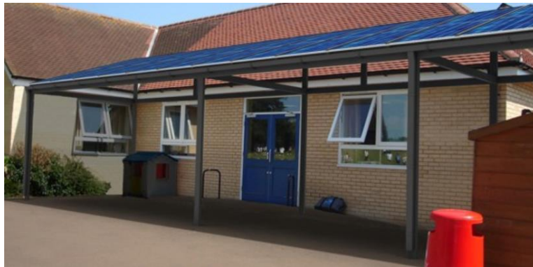
Solar PV canopy (aluminium)
